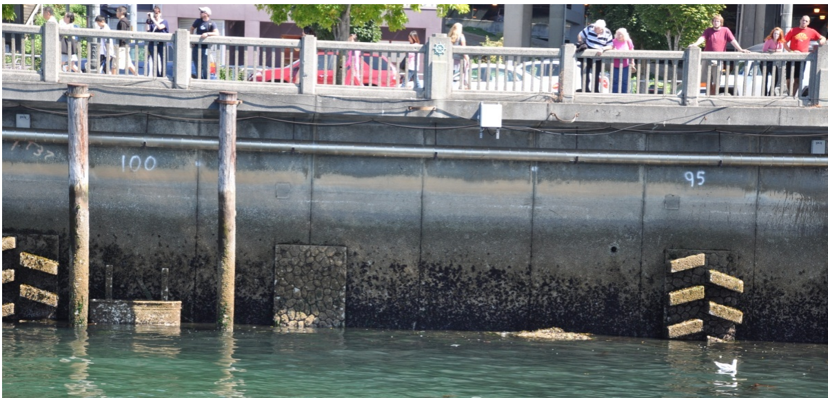
Habitat test panels on the Elliott Bay Seawall.
