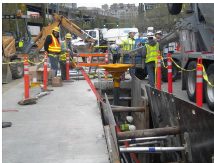
Utility duct bank excavation during Early Work on Alaskan Way.
