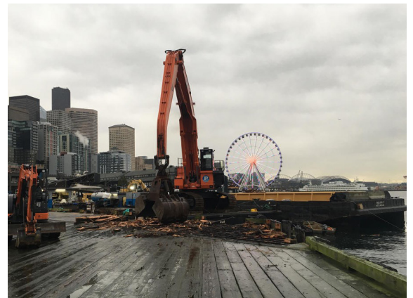
Example of pier deck removal.
