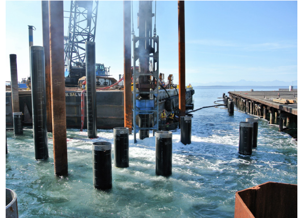
Example of pile driving.
