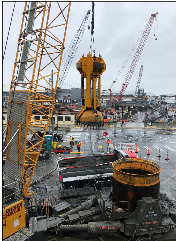
Example of drilled shaft installation.
