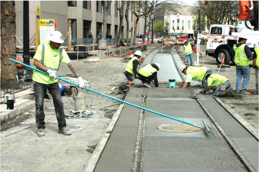
Raked tine concrete finish
