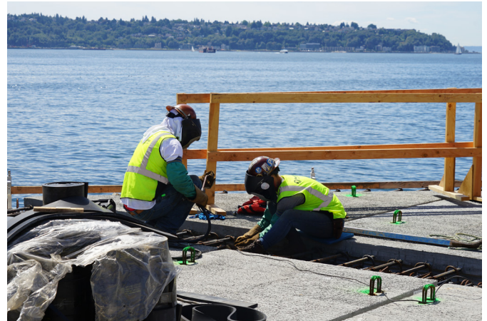
Workers secure pre-cast deck panels on Pier 62.
