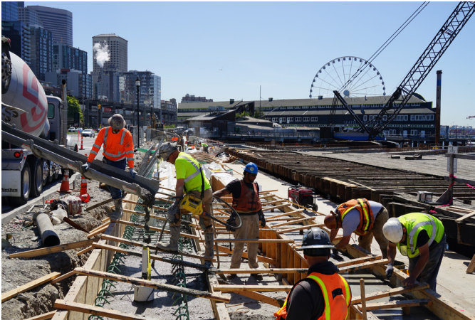
Concrete was poured into reinforced forms to create a temporary path along the west side of Alaskan Way, in front of Pier 62.
