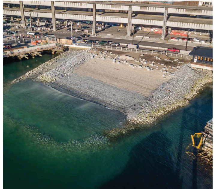
Rock installation was completed at the marine habitat enhancements.
