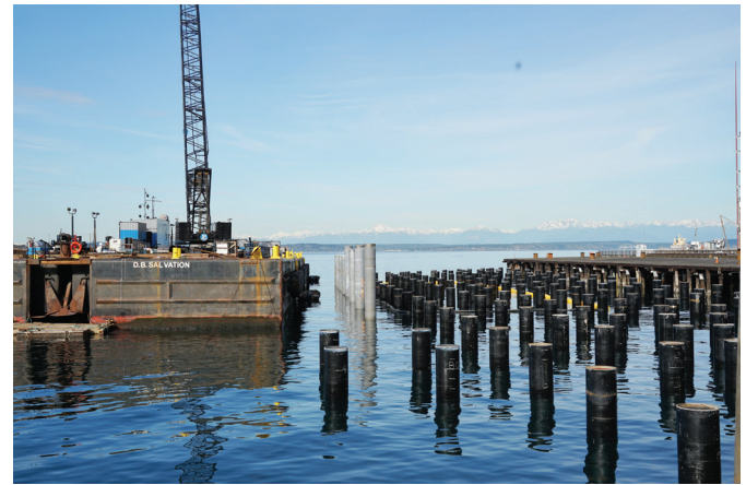
Pile installation continued at the Pier 62 Rebuild.
