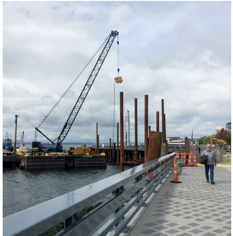
Test pile driving began at Pier 62 in September 2018.
