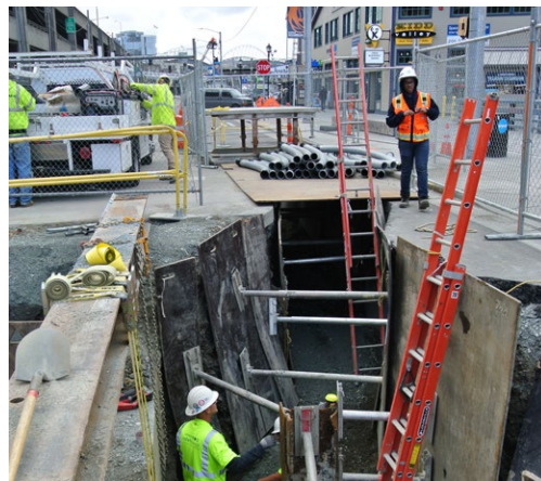
Preparation began for electrical vault installation between Spring and Seneca streets.
