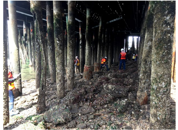
Crews inspected Pier 63 during low tide in June.
