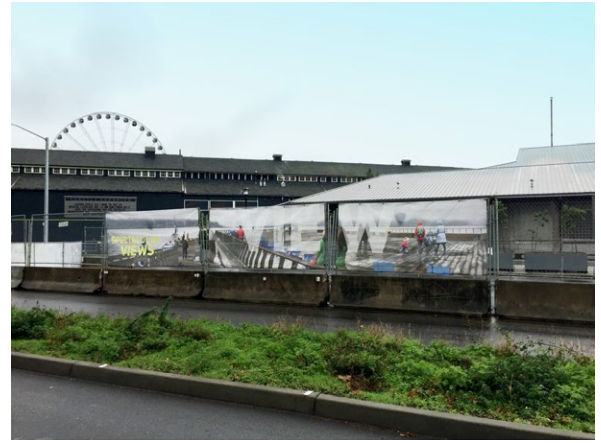
Banners showing the Pier 62 Rebuild were installed along construction fencing on Alaskan Way.
