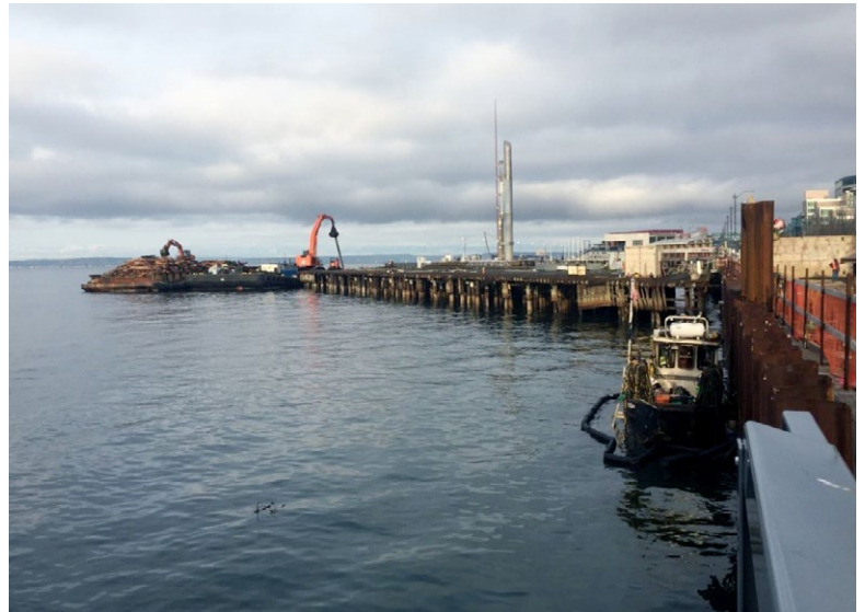
Crews completed demolition of Pier 62 in February.
