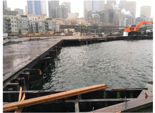
In February, crews completed demolition of Pier 62.
