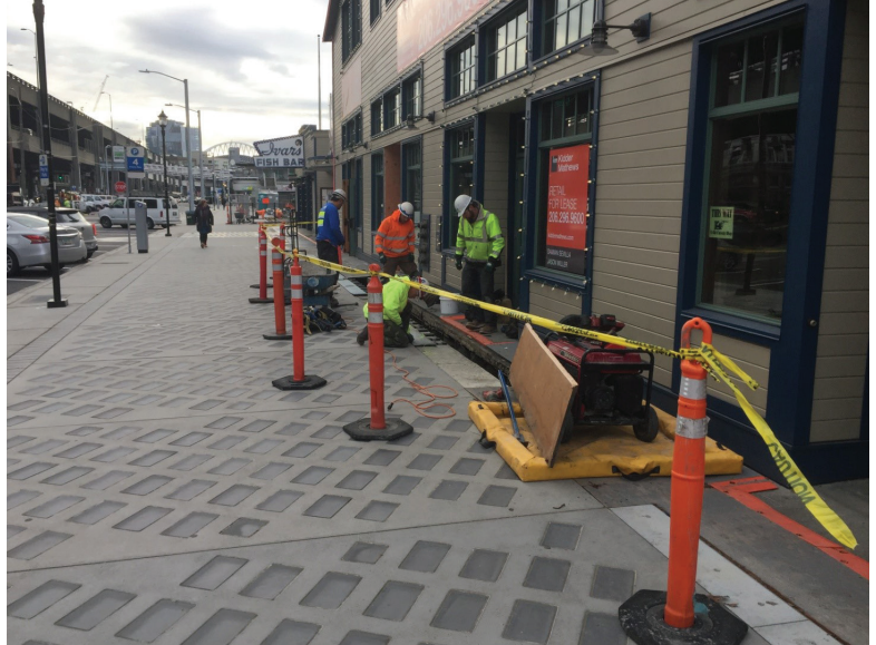
Seawall Project crews install light penetrating surface panels between Madison and Marion streets.
