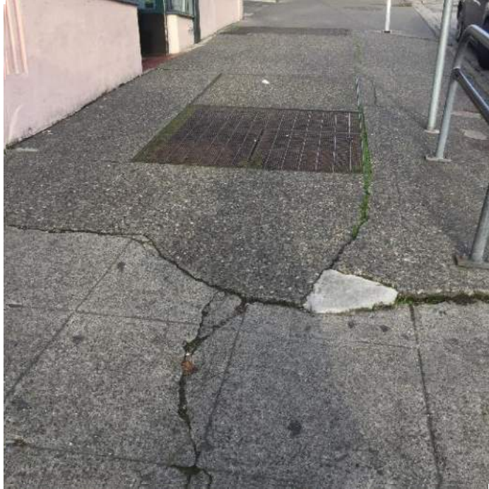
Poor Conditions: Cracked, uneven, patched, poor drainage
