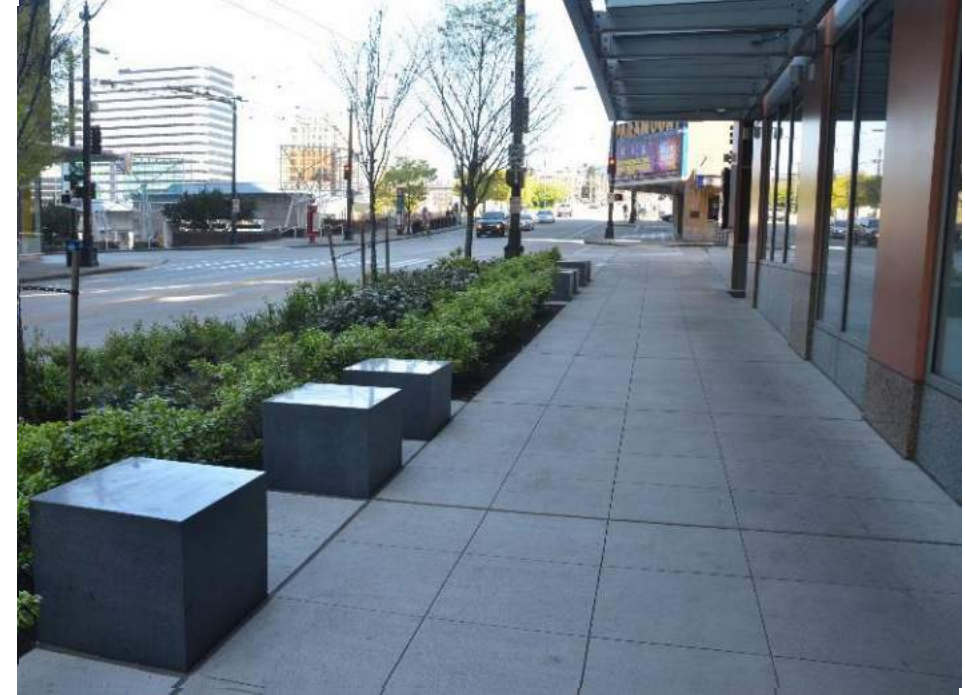
Good Conditions: Newer sidewalk, quality joints, smooth surface
