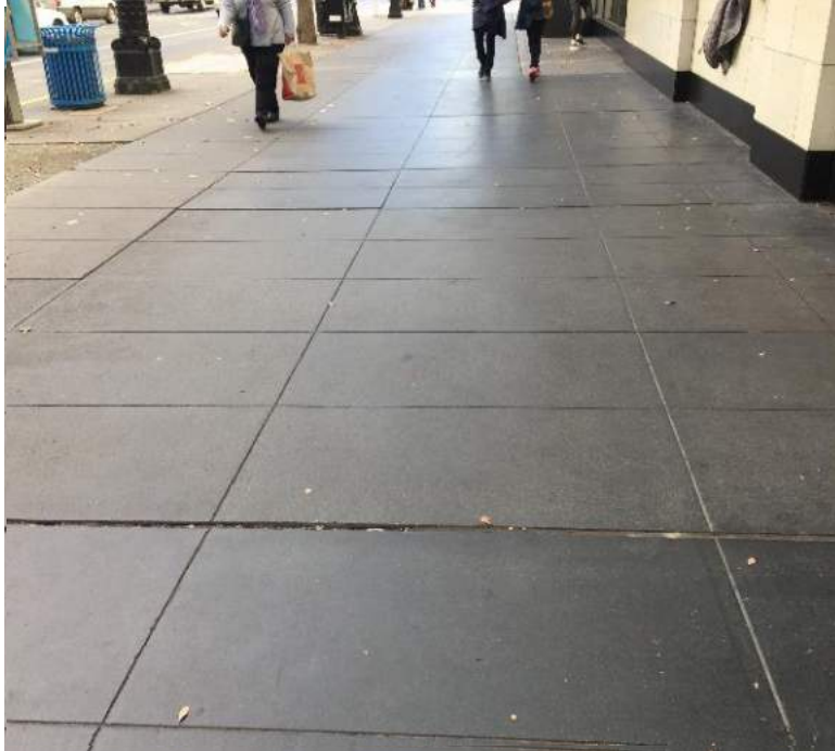
Moderate Conditions: Even surface, some patching, maintained joints
