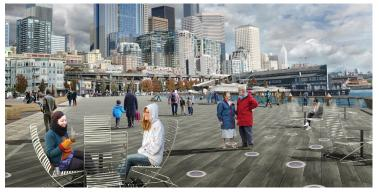
The rebuilt pier replaces old wooden pilings with steel pipe pilings and replaces the timber deck with a textured concrete deck. The circles in the decking are solar-powered lights.
