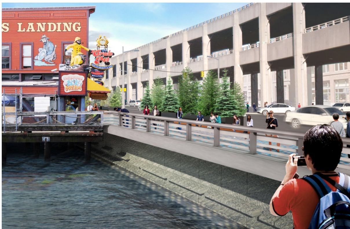
Rendering of the seawall final condition with textured wall face panels
