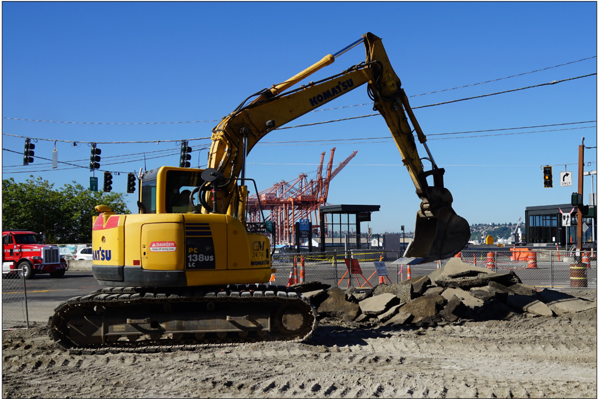
Example of roadway removal.
