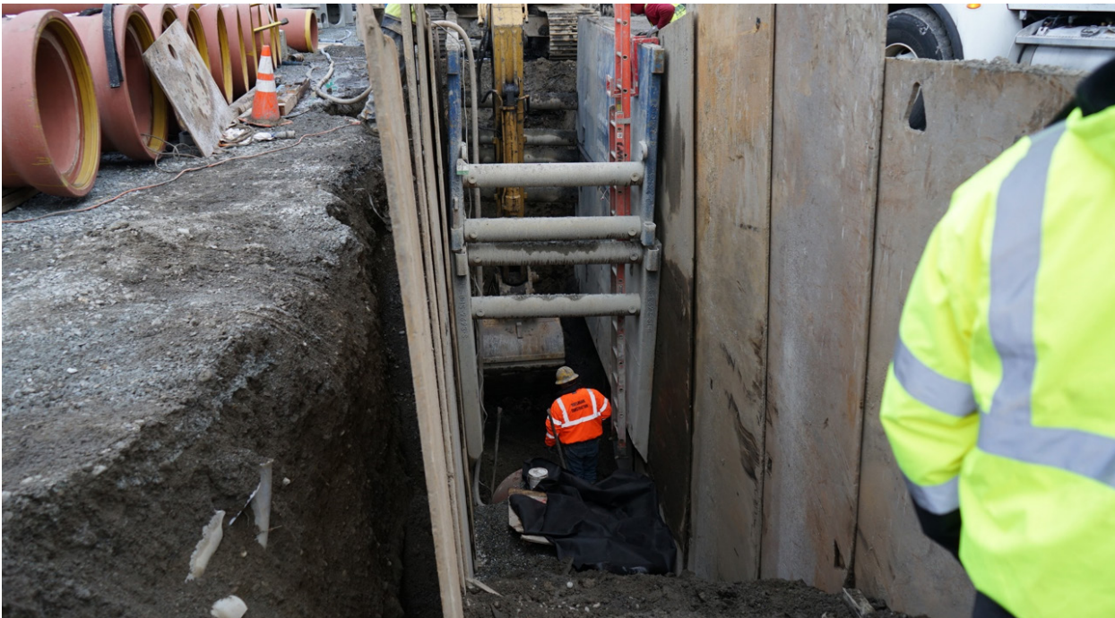
Example of sewer main installation.
