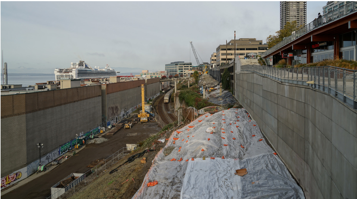
Photo of new work area and site of future Elliott Way.
